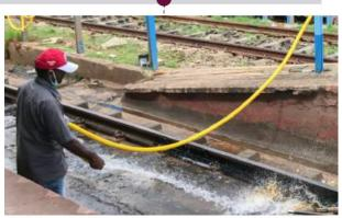
Pick up solid waste from tracks using scooper and put it in a bin; wear gloves and mask. Push excreta into drains using hose pipe (fitted along the tracks).
