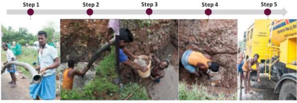
Machines and workers arrive at the location of the blockage. Diagnose issue, plan action, check for safety using rudimentary mechanisms. Attempt to use machines (suction, in this case), but have to guide the hose manually.
